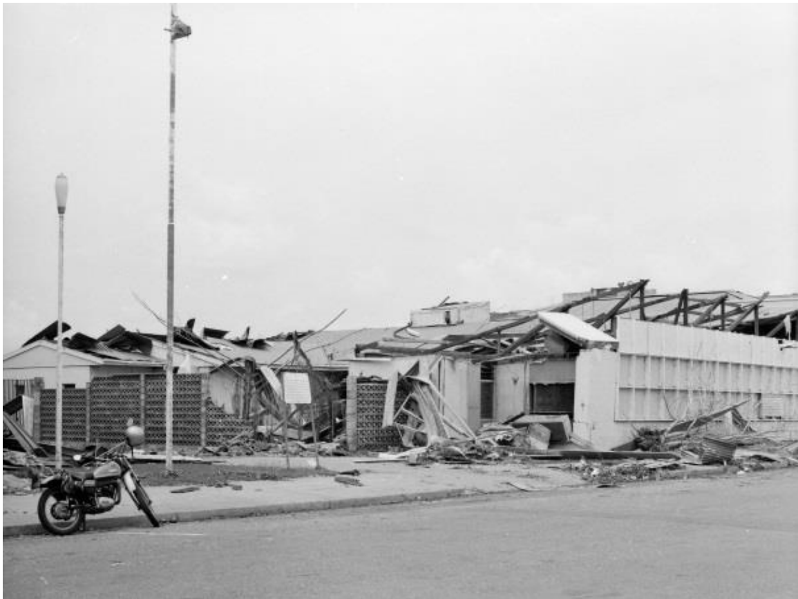
This view is from outside Block 2 looking at the Member's garden (left) and the PABX rooms (right).
