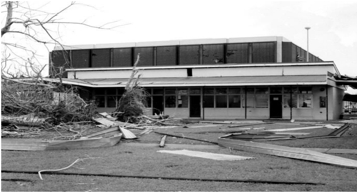
The Staff room (left) offices of the Clerks (center), Reception (right). The mailna trees near the offices were easily stripped of their leaves and uprooted by the cyclone. The building at the near the Chan Building, also known as Block 8 is where the Executive Members worked.
