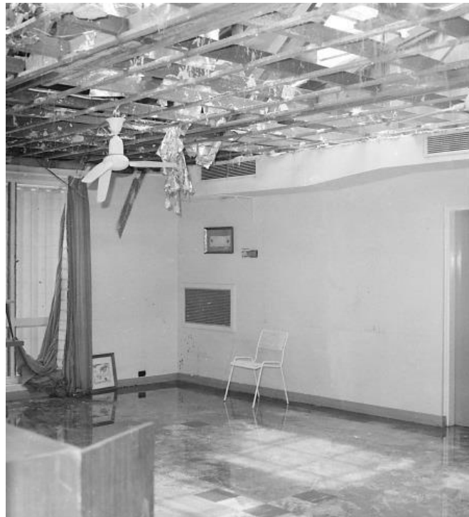
Inside the Members' Bar after the initial clean-up.
