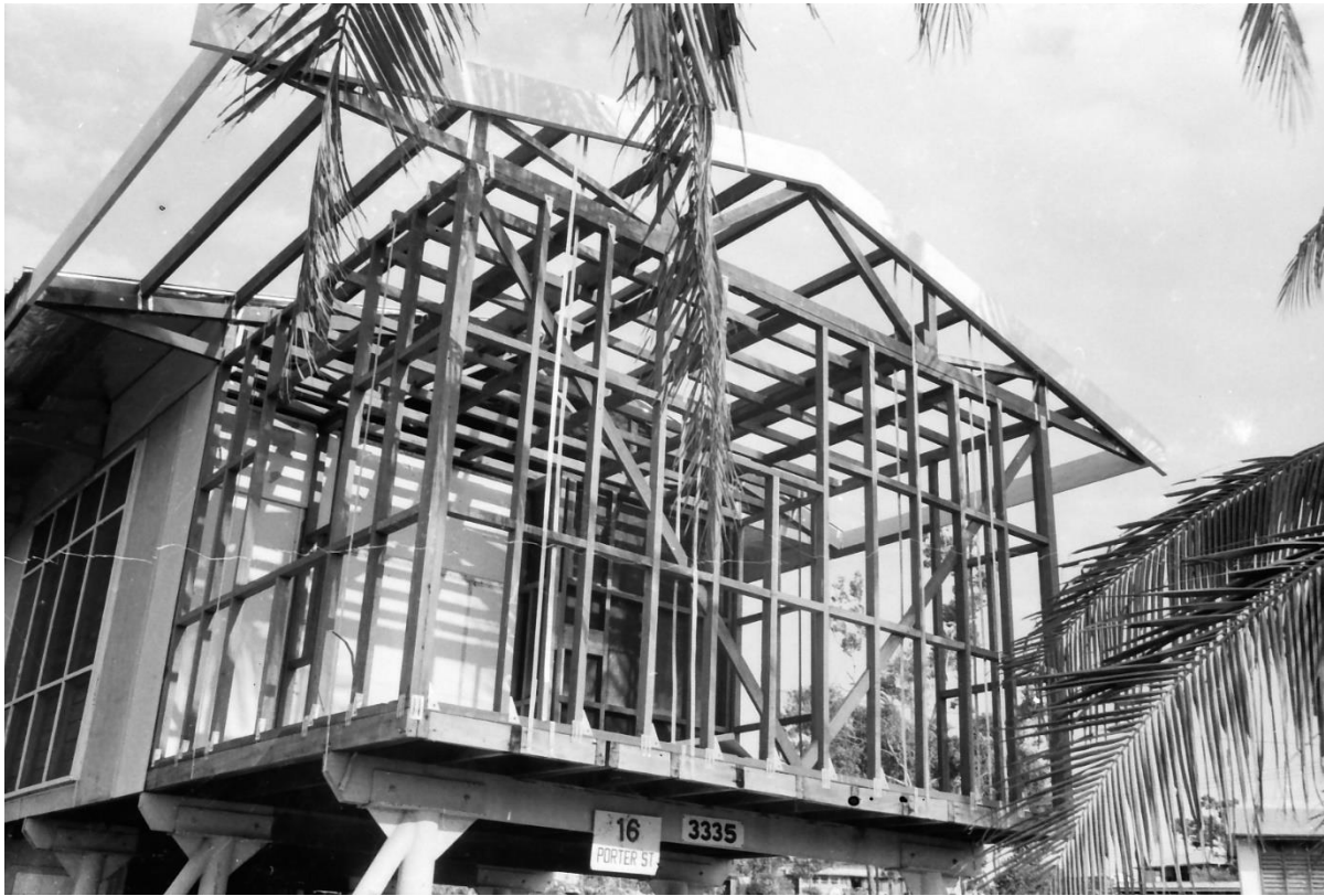
The construction of the main bedroom.
