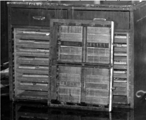
The left side of the picture shows a chase with 8 pages of Hansard . The printery had two compositors' imposing stones.
