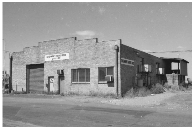
Prior to the occupation of the building the air-conditioning was serviced and stabilised.
