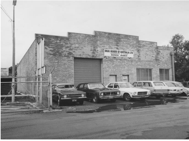
Early December 1974 – site chosen to accommodate the Government Printing Office while a new Printery was planned.
